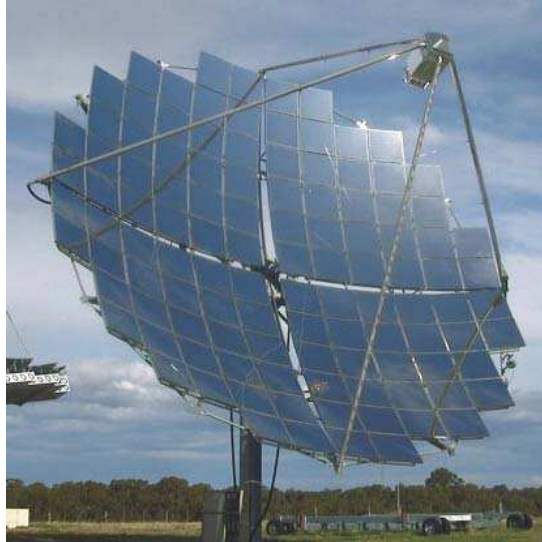
Figure 30. Solar Systems 20 kW CPV dish (NREL, 2007c).
