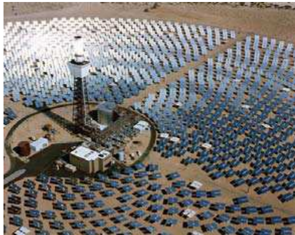
Figure 35. 10 MW Solar Two power tower system (NREL, 2006).
